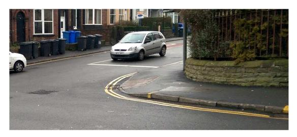
Although the proposals include for relocation of this crossing, the provision of the full-height replacement kerb face would still leave an excessive footway gradient falling towards the carriageway.
